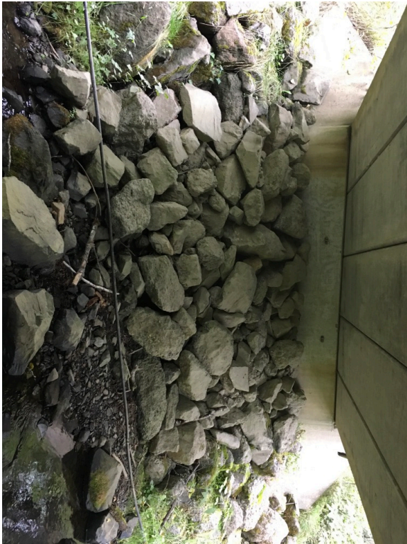
Right Bank Abutment when facing downstream
